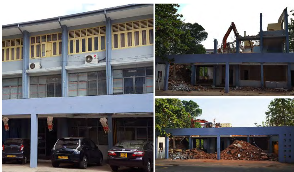
Figure 77: Old building of NSACP demolished in 2016
